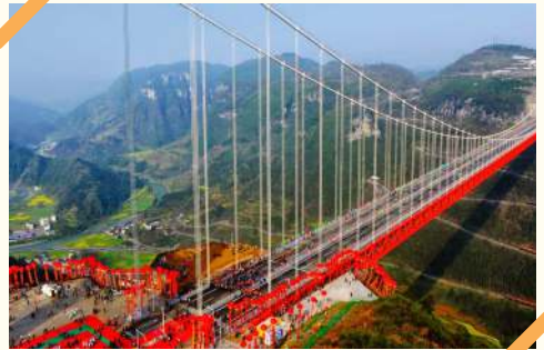
Baily Bridge (Ladakh) World's highest bridge
